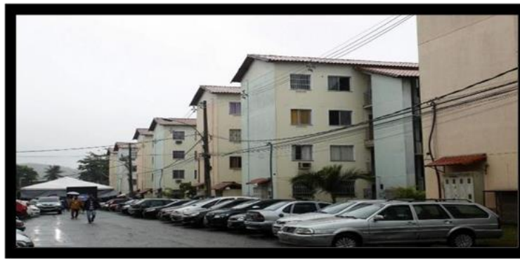
Figure 2. Courtyard at Destri condominium.
